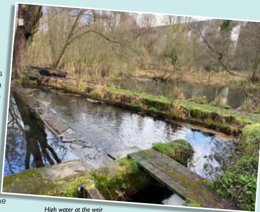
High water at the weir
