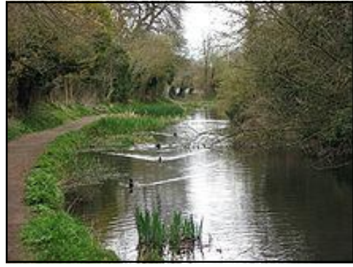
Disused section of the canal near Wendover
